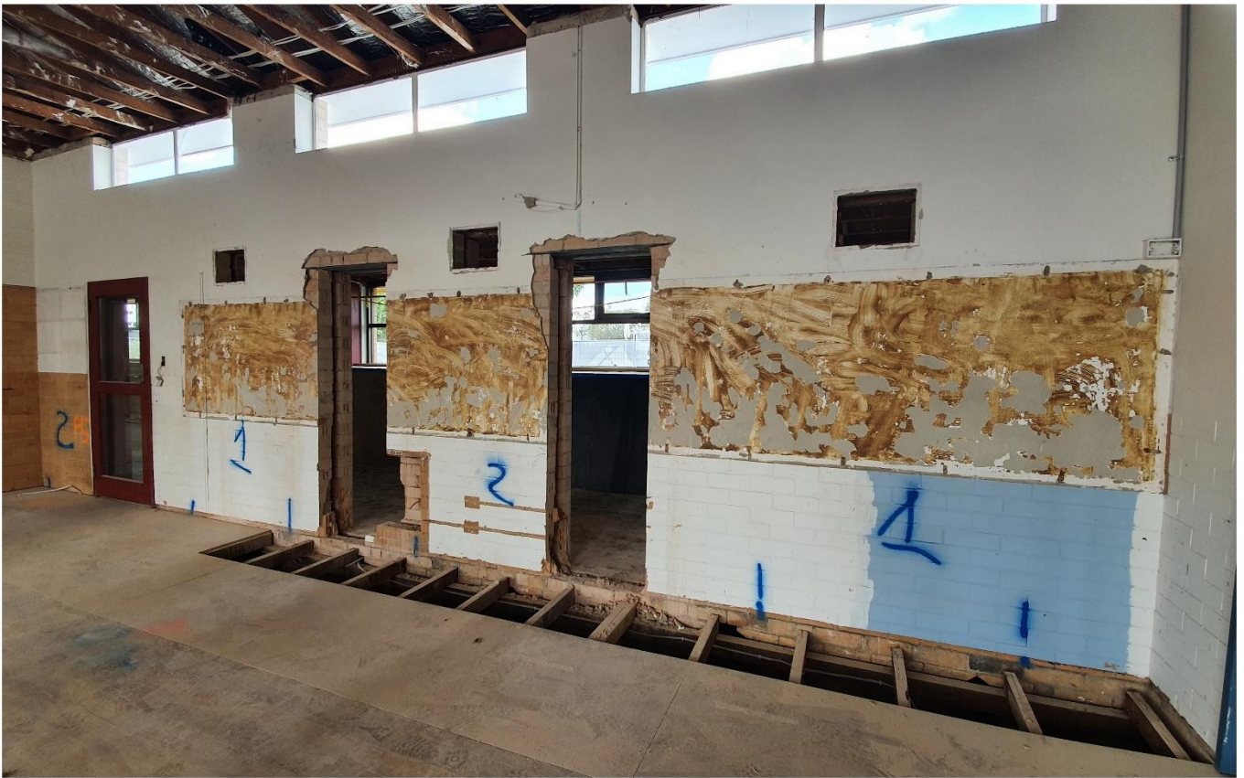
Roof and Floor Repair & New Corridor Window Openings
